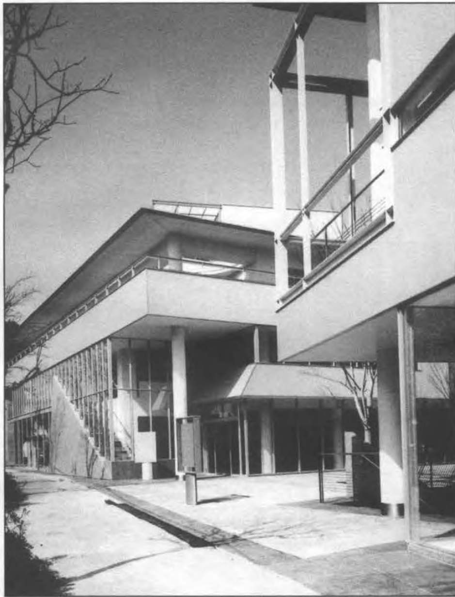
Fig. 11: View along Kyo Yamate Avenue (Phase VI). (Source: Maki and Associates, On Maki Architecture/Maki on Architecture , Tokyo, Fumihiko Maki Traveling Exhibition Executive Committee, 2001, p. 22, courtesy Toshiharu Kitajima).
